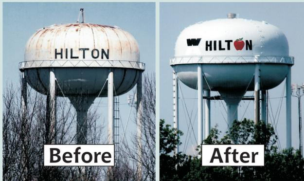
After 4,500 man hours of labor over the course of 4 months, using over 900 gallons of paint inside and out, the water tower project is finally complete!
